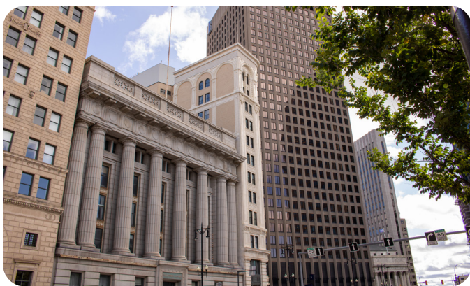
The Millennium Centre at 389 Main Street is the birthplace of Winnipeg's heritage movement
